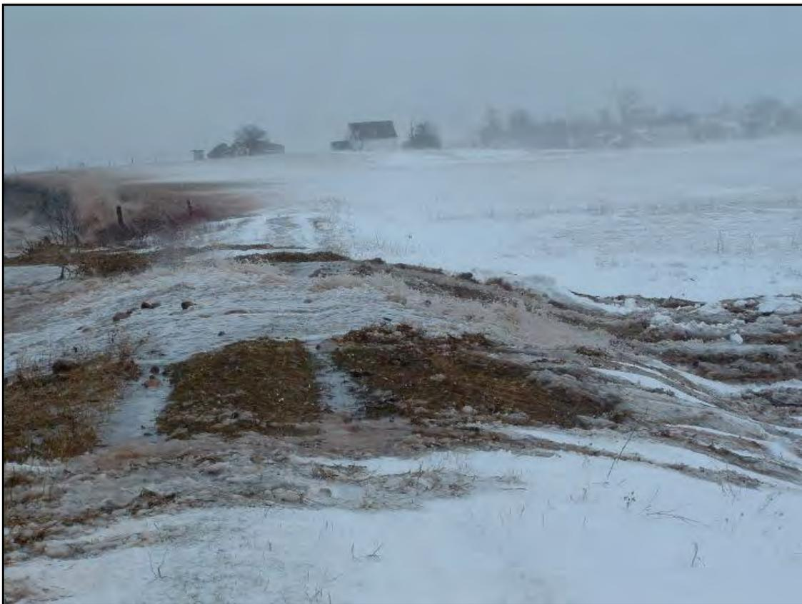
Figure 3: Storm impacts on Feb 1, 2006 at the Avonport Dyke. a) storm waves battering marsh; b) storm surge reached upper limits of dyke and dyke overtopped. Photo by T. Hamilton, 2006.
