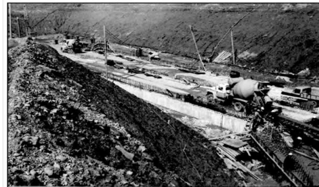
Construction of the dike (bottom) and aboiteau (top and right)
