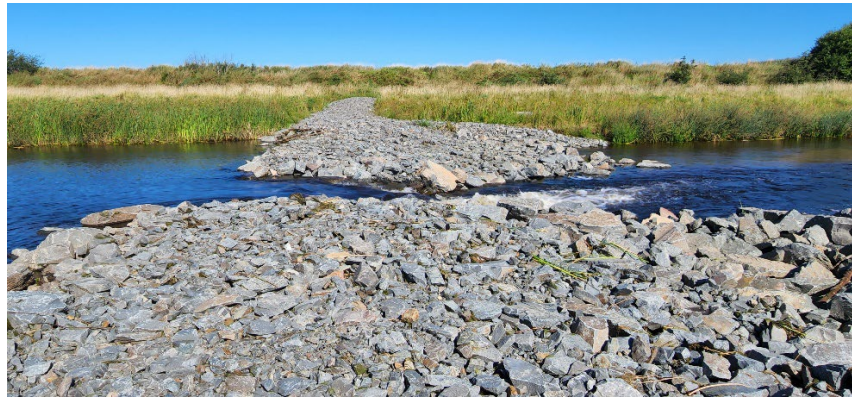
Figure 15: Martock fish habitat offsetting project - partial dam near T7–T8.
