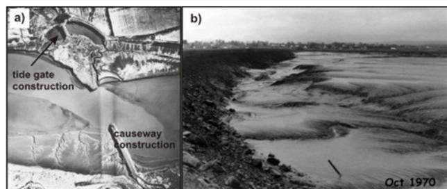
Figure 2: a) Rapid development of mudflat downstream of the Petitcodiac causeway in 1966, keeping pace with construction. Note dry land construction of tide gates; b) Rapid infilling of sediment adjacent to the Windsor causeway in Nov 1970.
